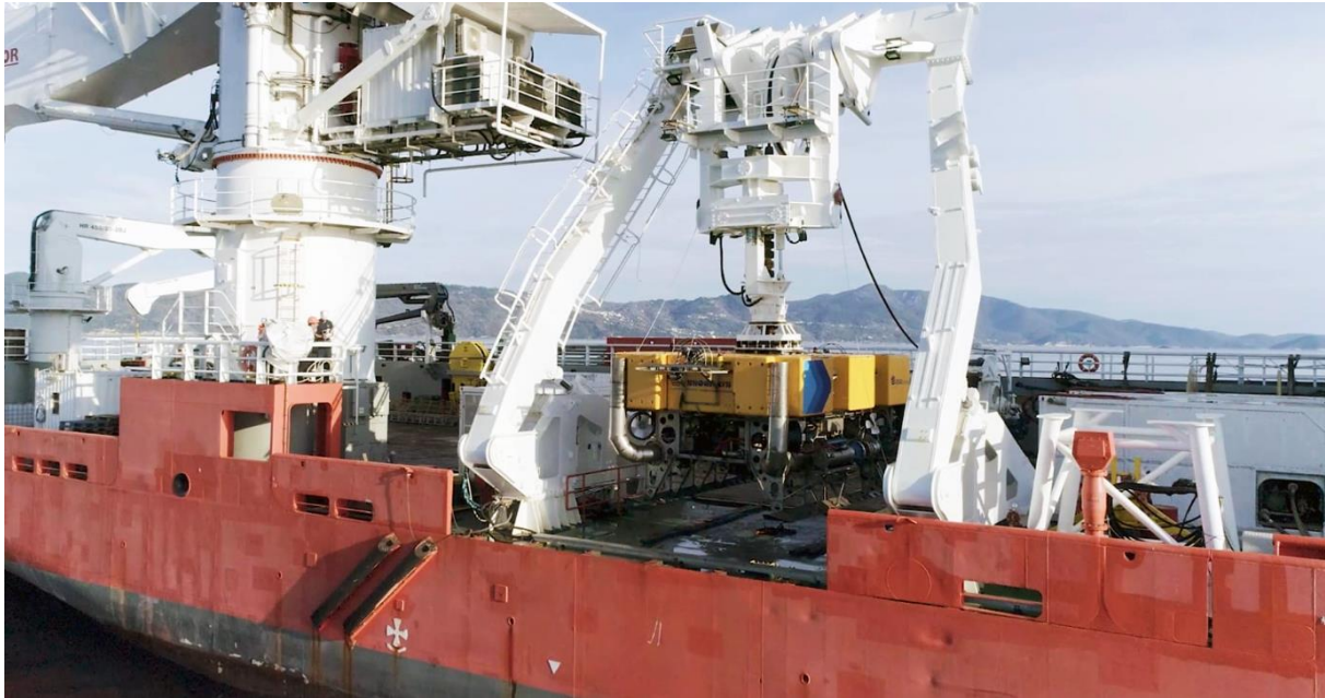
Figure 25: AssoJet III MK2 Jet Trencher
